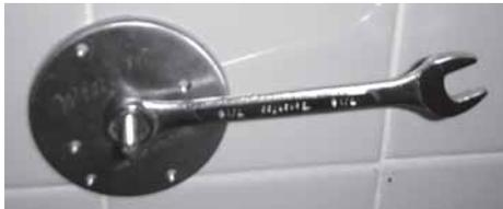
15. Pull on the bolt and tighten the nut by hand.
