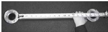
1. Verify the length of the grab bar, by measuring from the inside of one grab bar flange to the outside of the other. This should give you the proper dimension.
