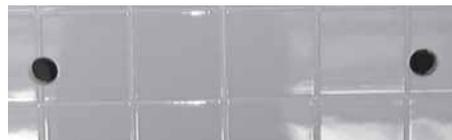
7. Picture of a ceramic tile wall with 2, 1-1/4" (30mm) holes –Ready for WingIt™ Installation.
