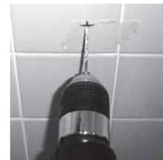
2. Use a 1/8" (3mm) drill or punch to make a starter/pilot hole. Once the first pilot hole is drilled check your measurement to
