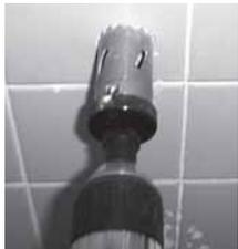
3. Carefully drill a 1-1/4" (30mm) hole in the wall precisely at the center point where each grab bar flange will align. In Ceramic Tile a piece of masking tape over
