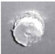
6. Then carefully finish the 1-1/4" (30mm) hole through the drywall. Do not push the drill. Allow it to cut, keeping the drywall intact behind the wall.
